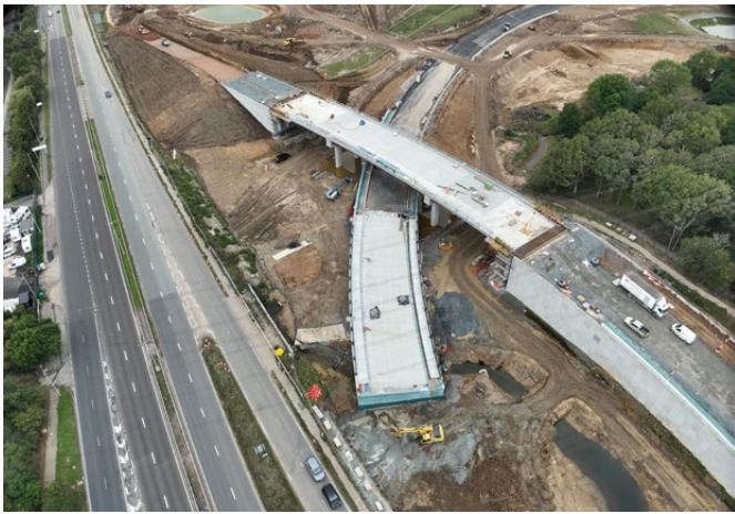
Progress of M25 junction 28 scheme.
