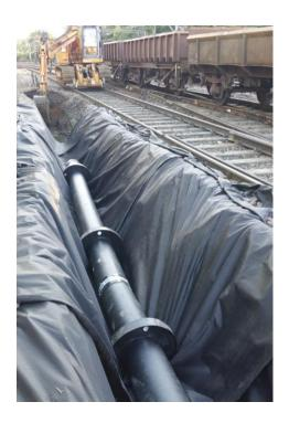
Example of an acoustic shroud, used to reduce the noise of our piling works, along with a photo of the current drainage works being undertaken.
